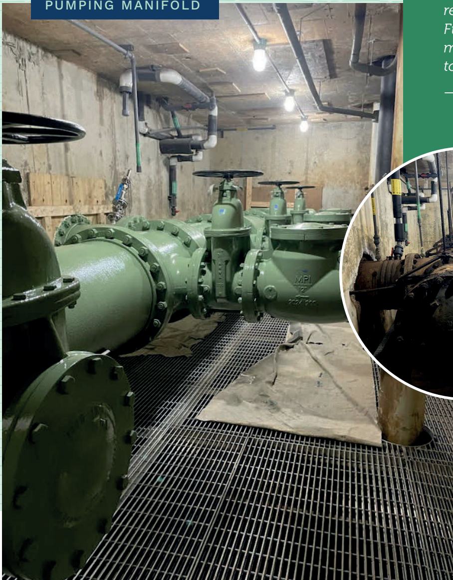
NEW RAW WATER PUMPING MANIFOLD
